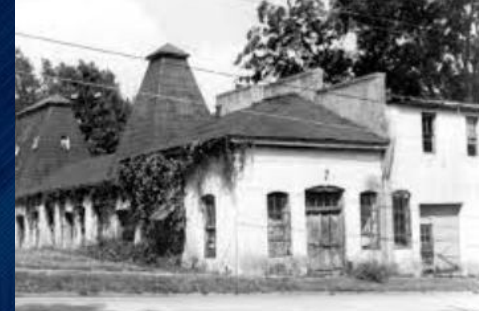
The Old City Waterworks sits idle (1974)
