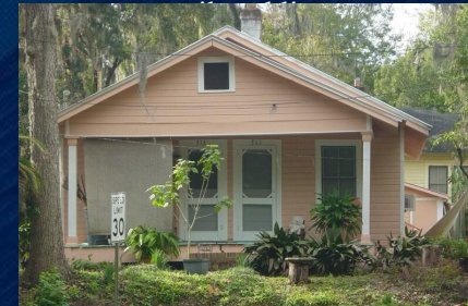
Some homes from Smokey Hollow were not destroyed, like this one on Lafayette Street, built in 1926.
