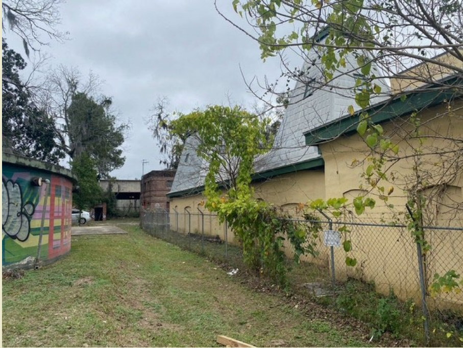
Prior to adaptive reuse: building exterior
