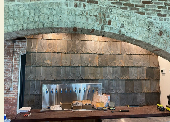
Original brick, tin roof tiles and cedar joists
