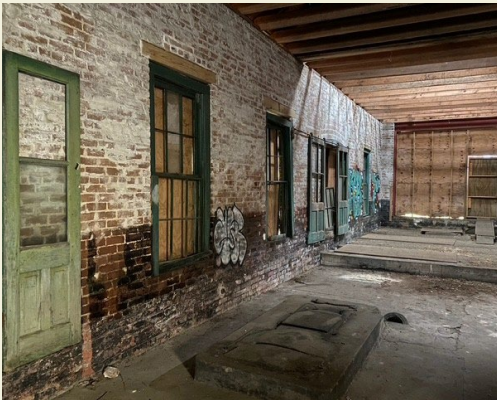
Historic doors and windows
