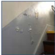
Lead-based paint was found throughout the building prior to being addressed.
