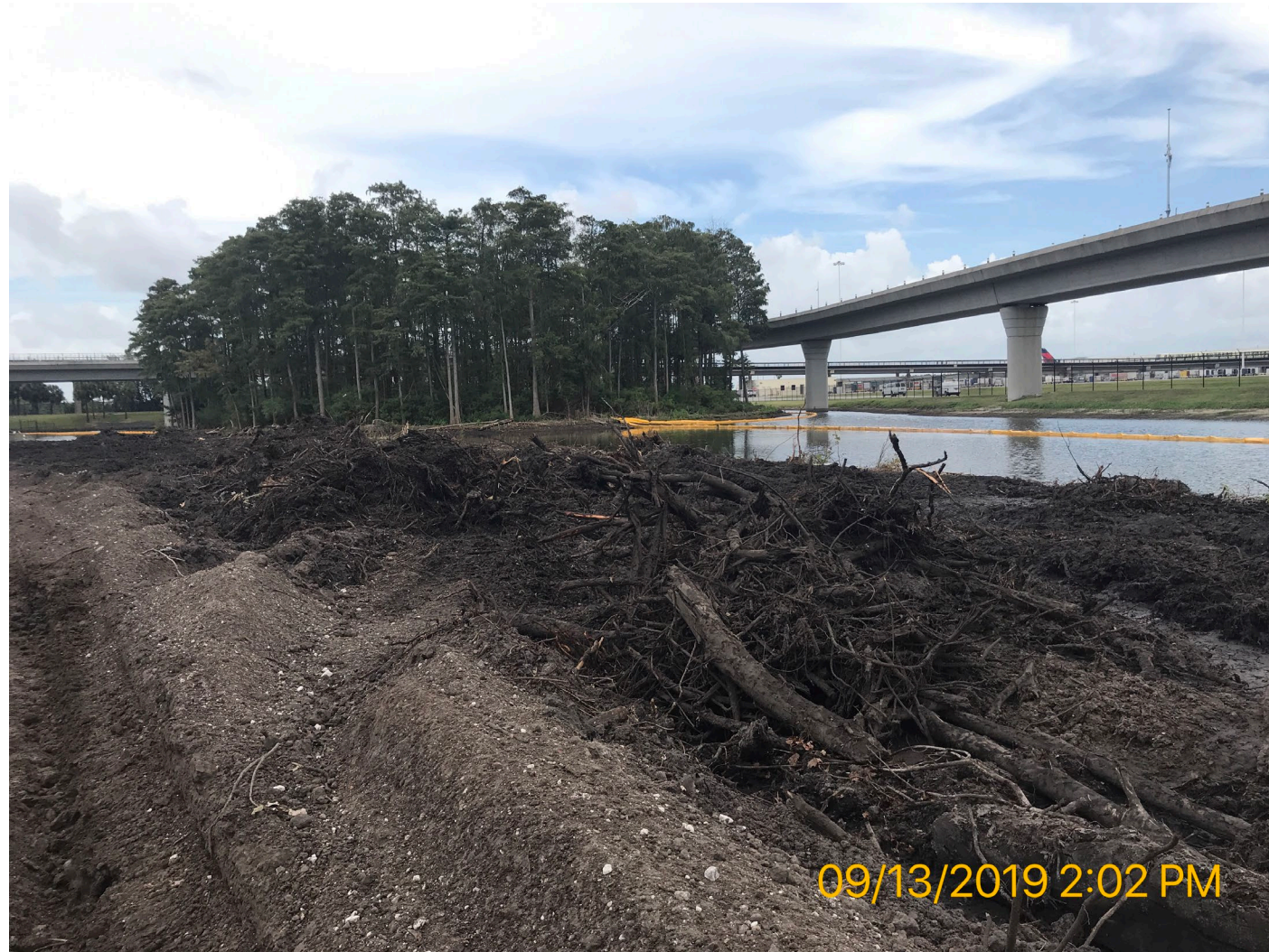
Clearing and Grubbing
