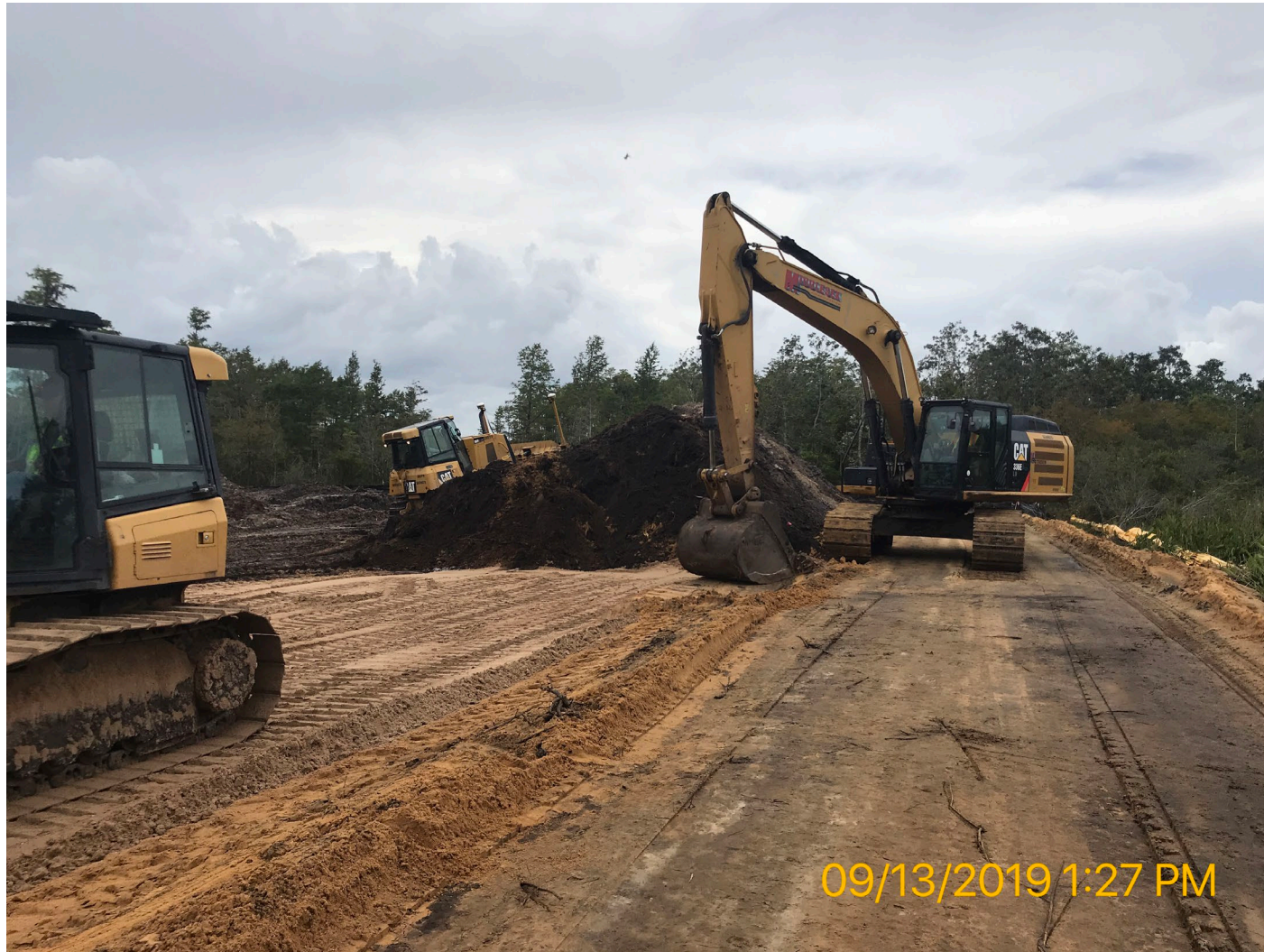
Embankment Construction
