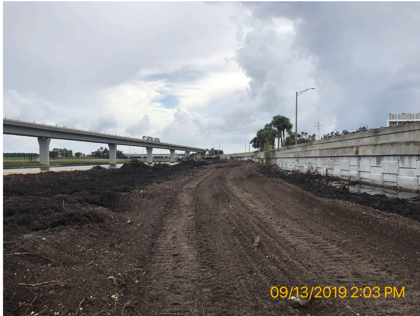
Clearing and Grubbing
