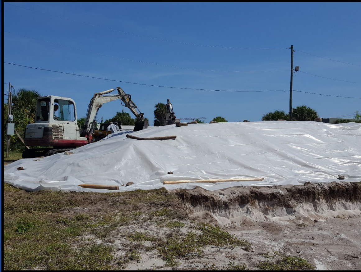
Excavated Soil Cover Until Disposal
