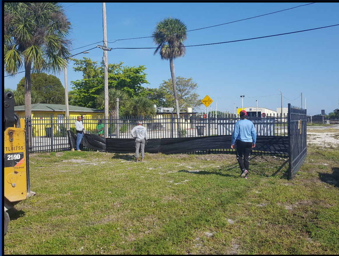
Prior to excavation-putting in perimeter controls
