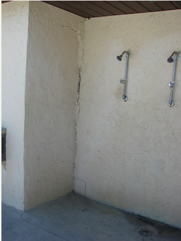
Pool house: cracks, outside shower area
